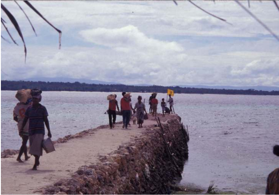
Plate 3-2: The under construction stone dock in Ohoislam (1996).
