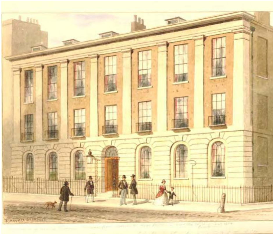
Figure 4.4 Arundel Street entrance of the Crown and Anchor tavern.
