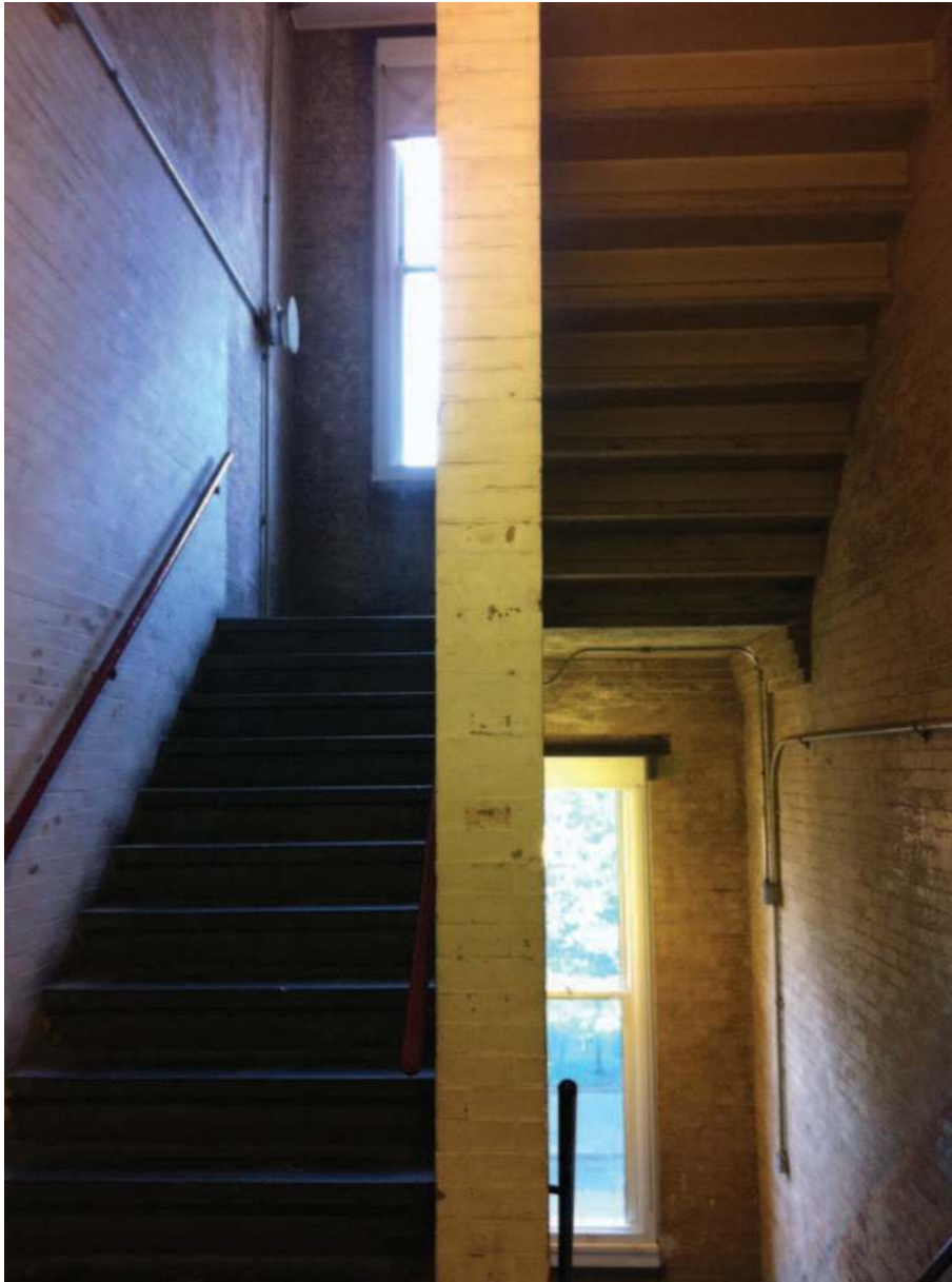
Stairs leading to the boys club.
