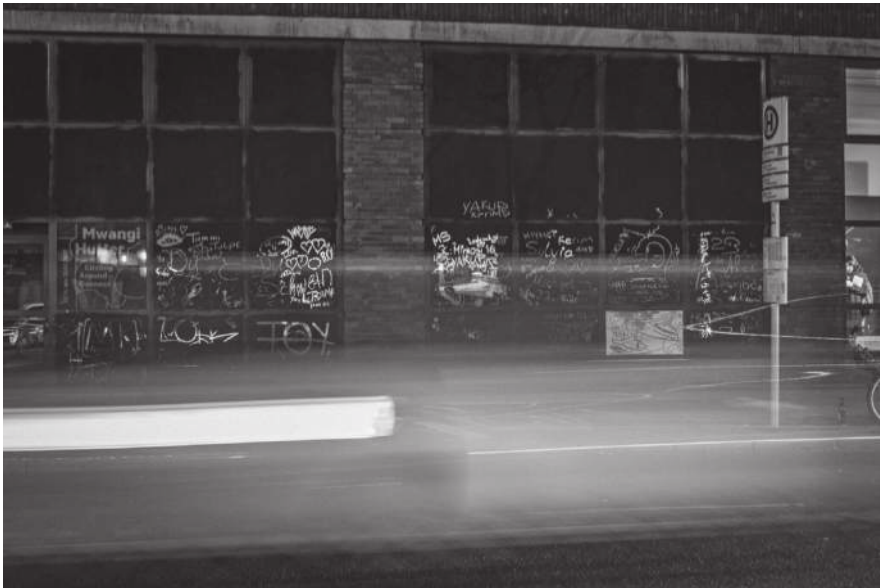
Fig. 10.2 View of the gallery membranes from Müllerstraße during the exhibition Circling Around Oneness (2016) by Mwangi Hutter, Galerie Wedding, © Fernando Gutiérrez Juárez
