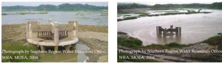
Figure 2. Shaft spillway pipe.
