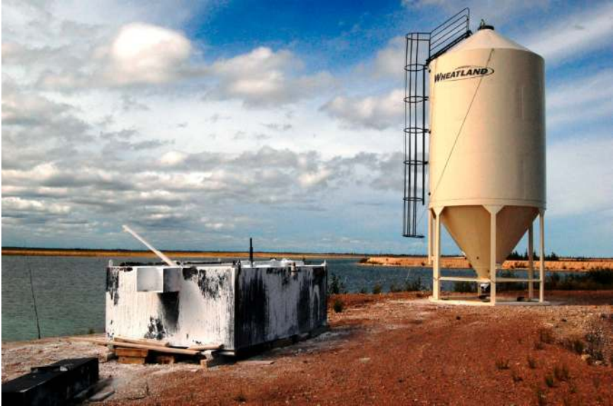
FIG. 11.2: Tailings area at the former Pine Point Mine, where overflow water is treated with lime to precipitate zinc. Photo by Arn Keeling.
