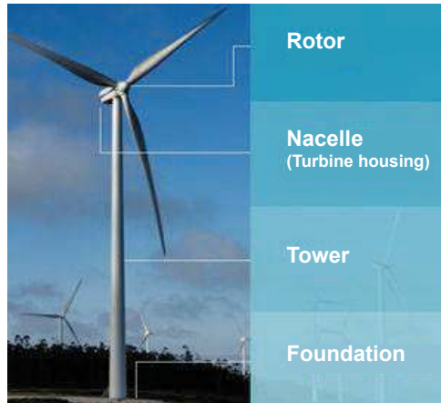
Figure 3. Major turbine parts docera.com/wiki.
