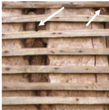
Figure 1. A traditional external tabique wall showing corncob as a filling material.
