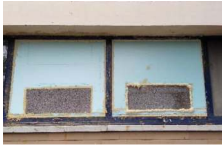
Figure 16. Thermal insulation test of CMU (exterior view). March 2014.
