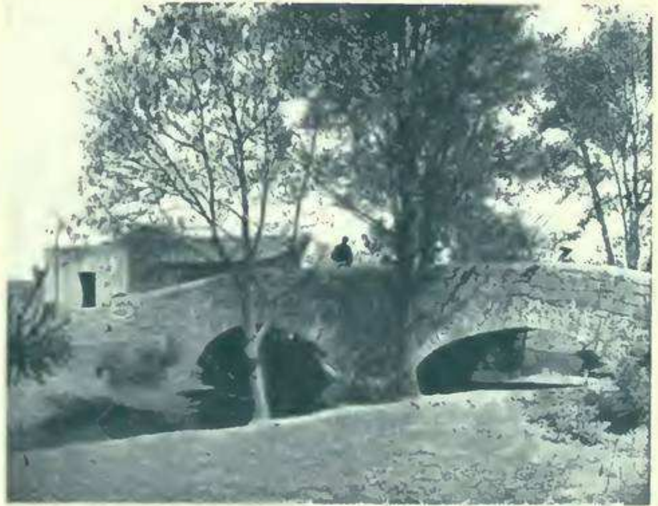
BRIDGE AT TEOLOVUCAN, STATE OF MEXICO.
