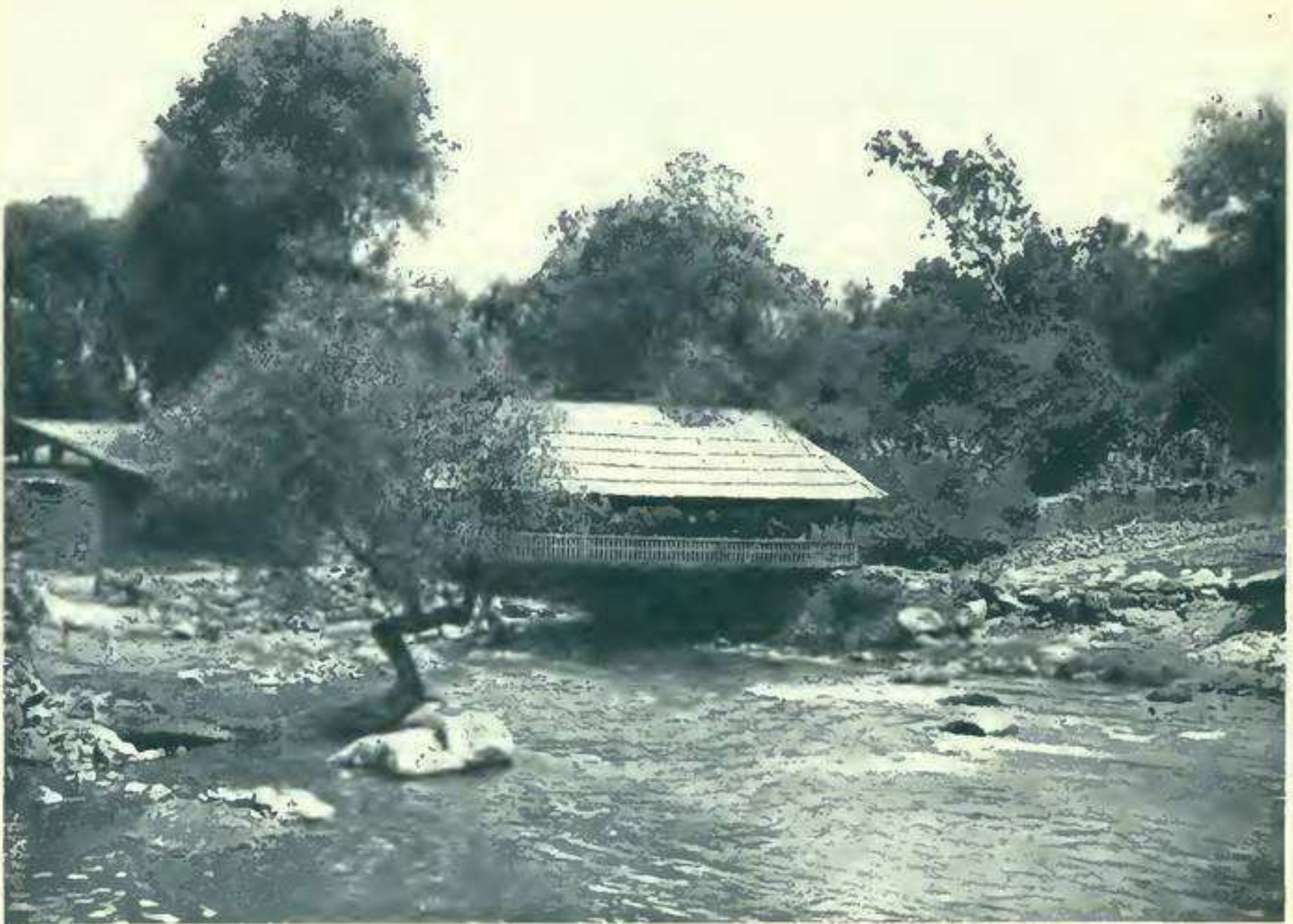
WOODEN BRIDGE AT URUÁPAM.
