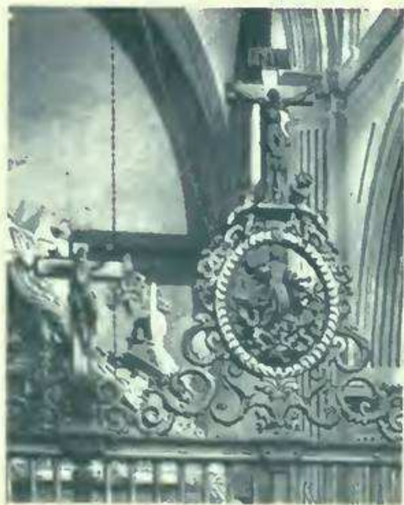
CATHEDRAL OF MEXICO: DETAIL OF METAL WORK ON CHOIR-SCREEN.
