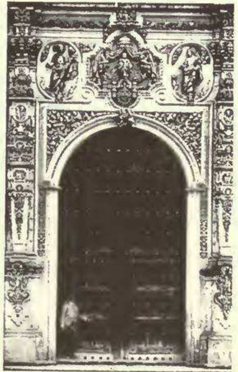
DETAILS OF ORNAMENT ABOUT DOOR OF CHURCH AT TEPOZOTLÁN.
