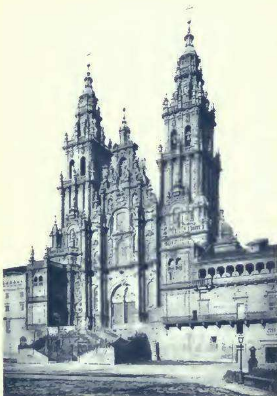
FACADE OF THE CATHEDRAL OF SANTIAGO DE CAMPOSTELA, SPAIN.
