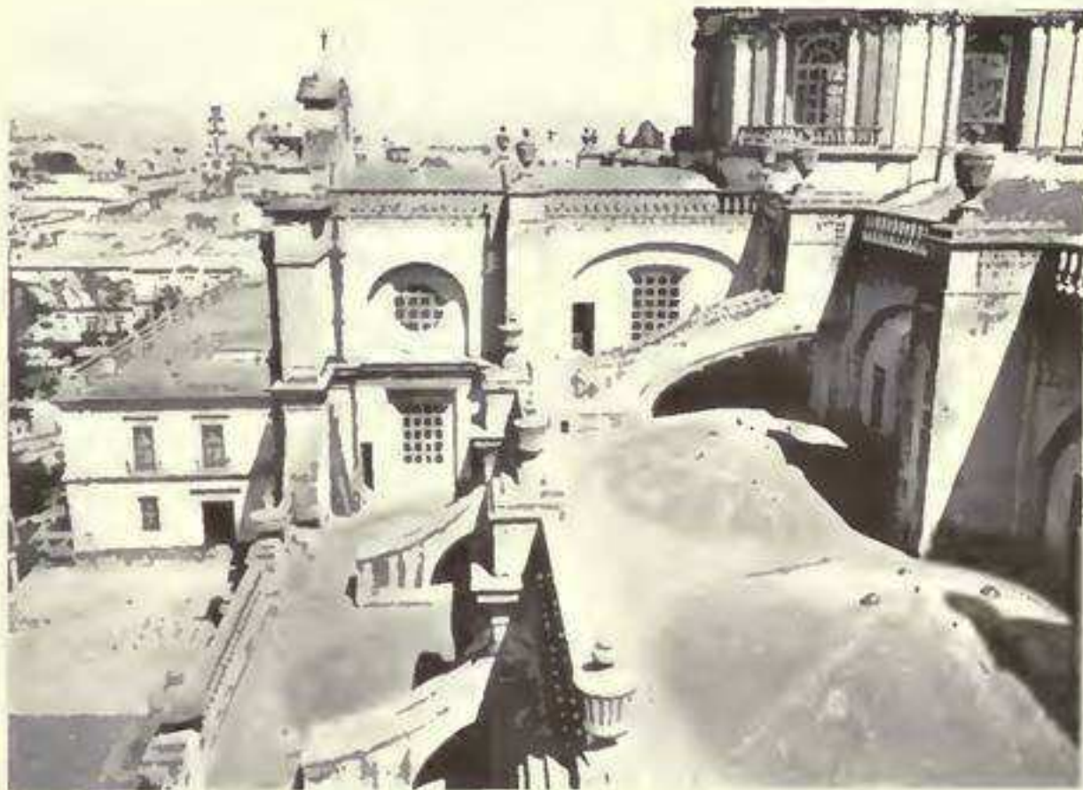
THE CATHEDRAL OF MEXICO: ROOF OF NAVE, TRANSEPT, WEST AISLE AND CHAPELS FROM WEST TOWER.
