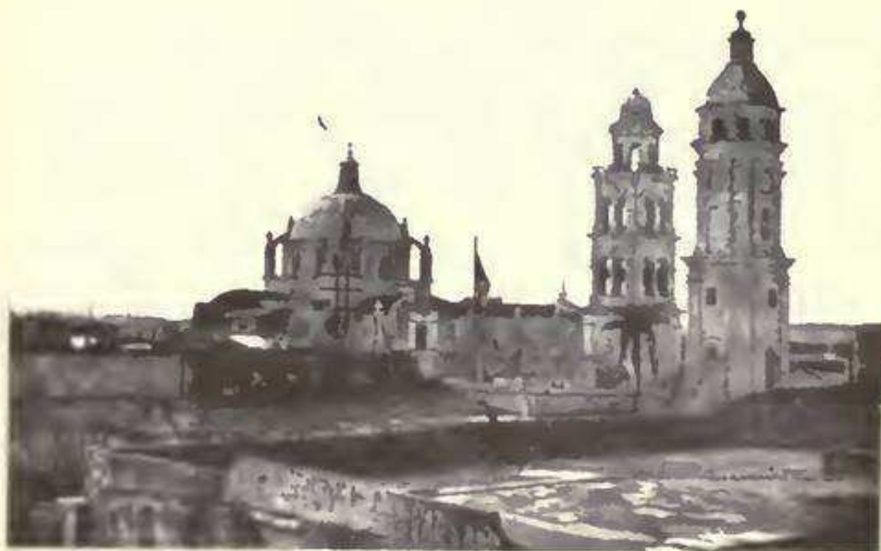
TOWERS AND DOME IN VERA CRUZ.
