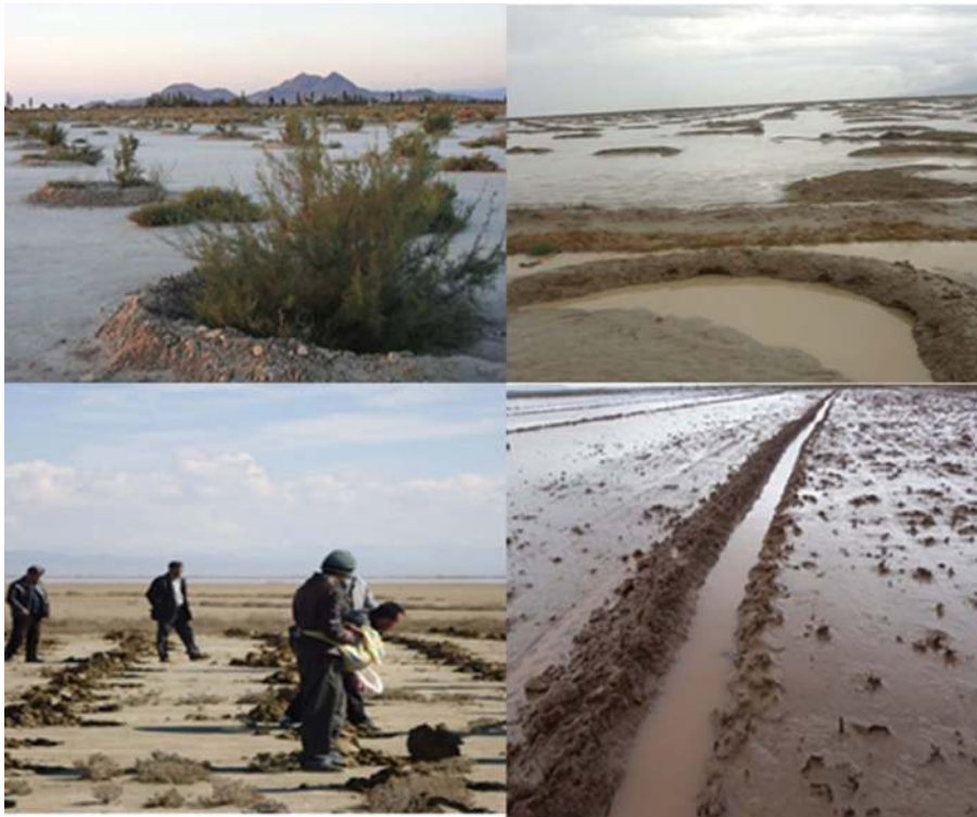
FIGURE 9.10 Surface runoff and sewage control operations in saline lands around Lake Urmia. (Source: www.ulrp.ir .)
