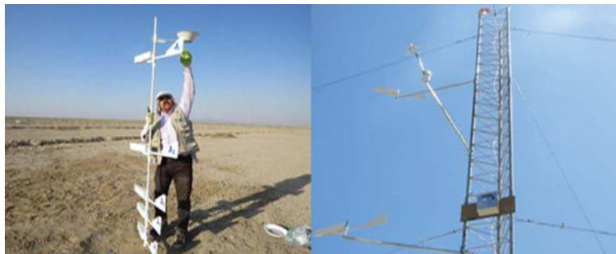
FIGURE 9.11 Construction of a quantification station of wind erosion and salt dust events. (Source: www.ulrp.ir .)
