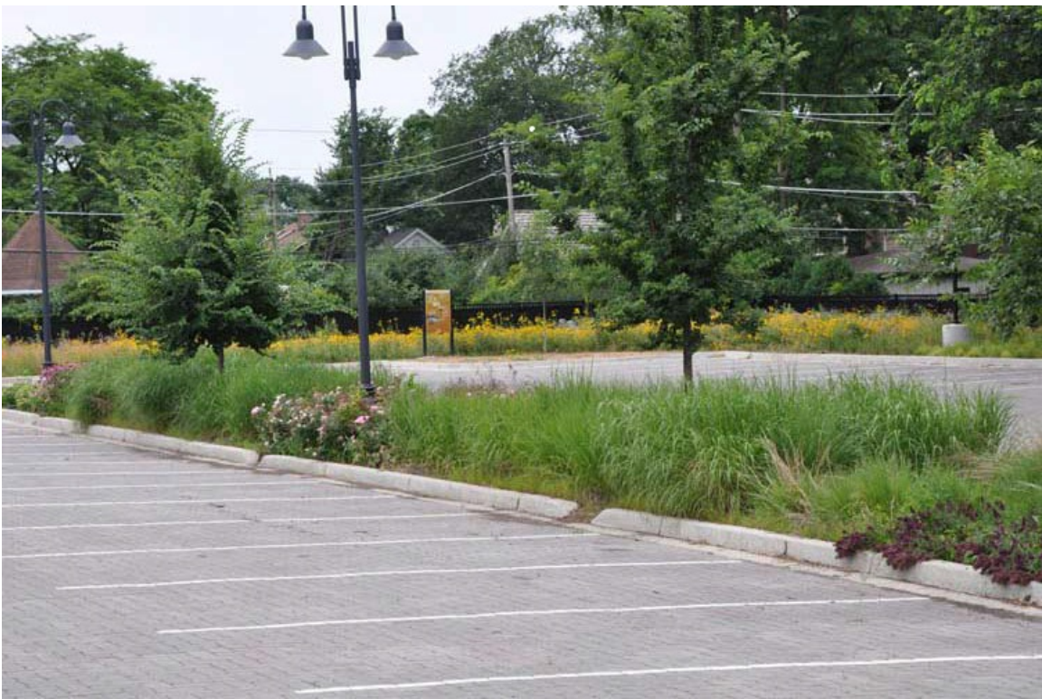
Figure 11.32: Permeable Paving & Vegetated Swales Permeable paving drains into a vegetated swale as part of Elmhurst College's (in Illinois) parking lot's "green" stormwater management system. Source: Jaffe, M., et al. (2010) (p. 587), Fig. 14, p. 117.
