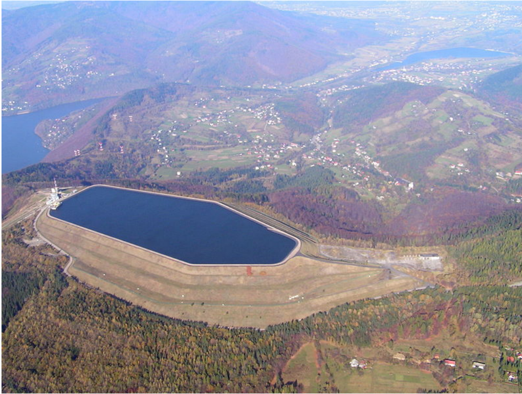
Figure 8.26: Pumped Hydroelectric Storage Upper storage reservoir for pumped hydroelectric storage, an established technology for storing large amounts of grid electricity. Source: Ongrys via Wikimedia Commons 85
