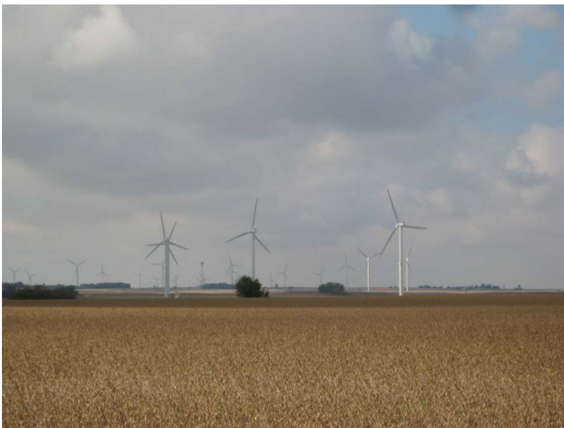
Figure 8.18: Twin Groves Wind Farm, Illinois Wind power is becoming a more popular source of energy in the United States. Source: Office of Sustainability, UIC 49
