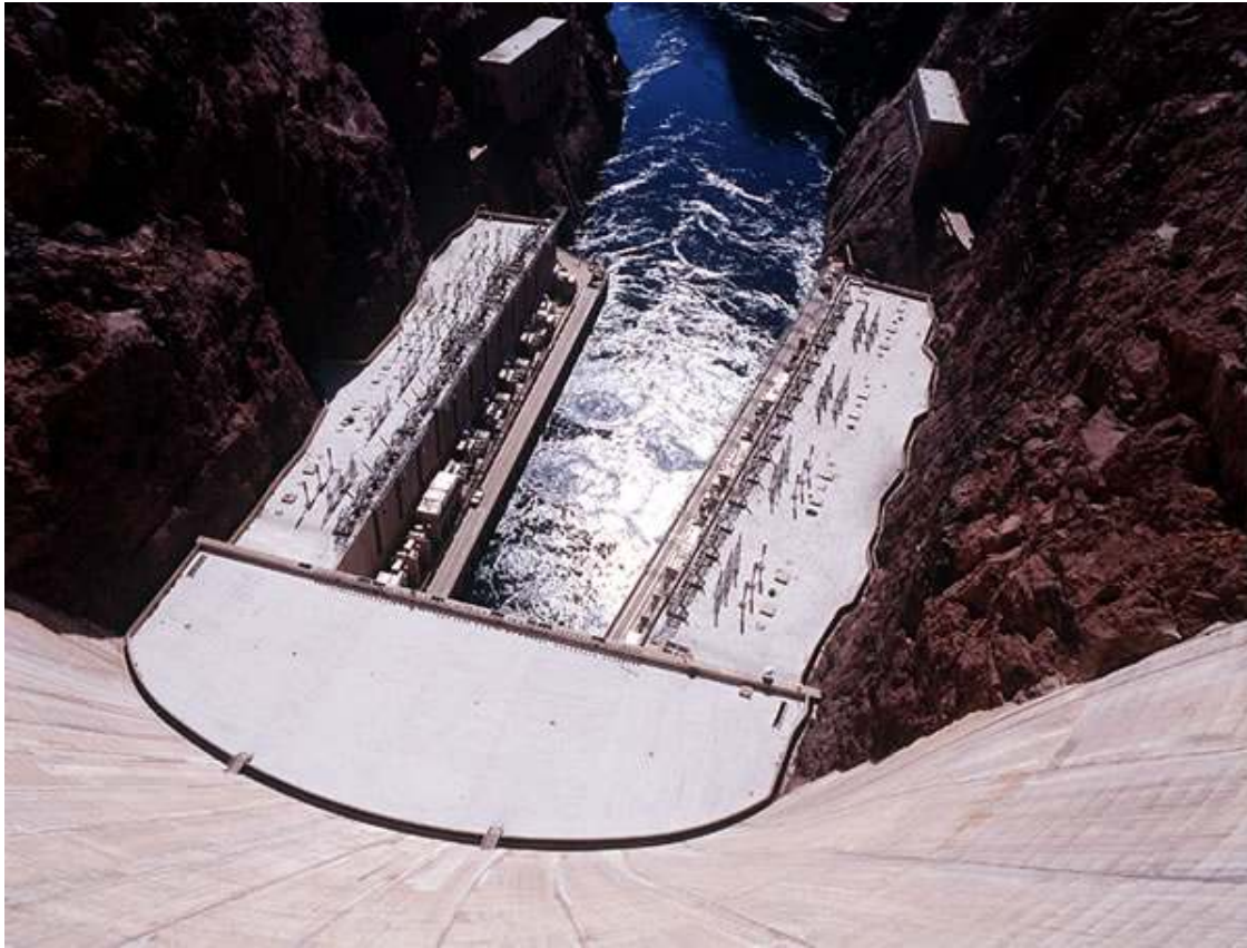
Figure 8.14: Hoover Power Plant View of Hoover Power Plant on the Colorado River as seen from above. Source: U.S. Department of the Interior 41
