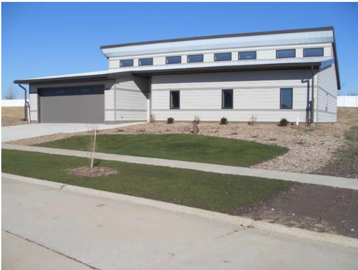
Figure 11.35: The Equinox House The picture of the house on a sunny November day shows the passive solar entering the clerestory windows. Source: ©2012 Equinox Built Environment Engineering; a division of Newell Instruments Inc. 130
