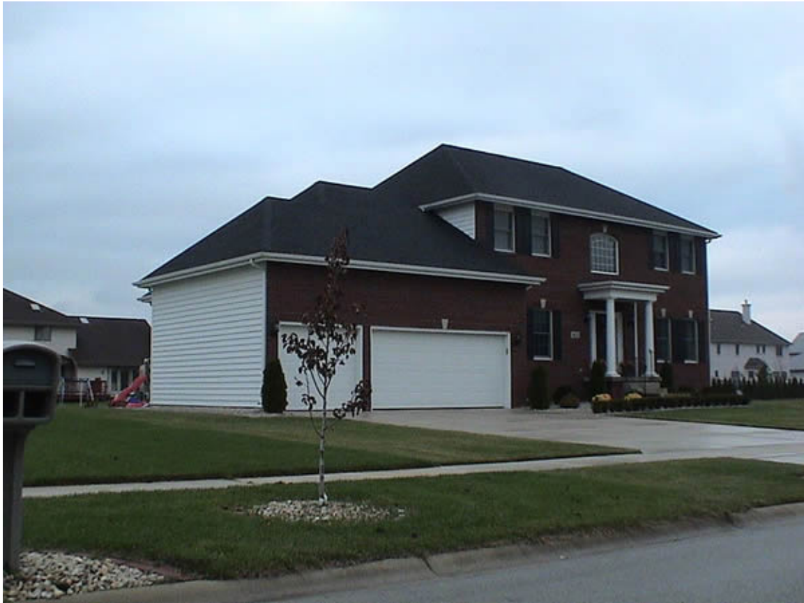
Figure 11.6: McMansions Home with large garage and short driveway depth taking up a large amount of street frontage. Also evident: several cheaply installed neoclassical elements, a brick facade, no side windows, and poorly proportioned windows on the front. Source: John Delano of Hammond, Indiana [CC0 26 ] via Wikimedia Commons 27
