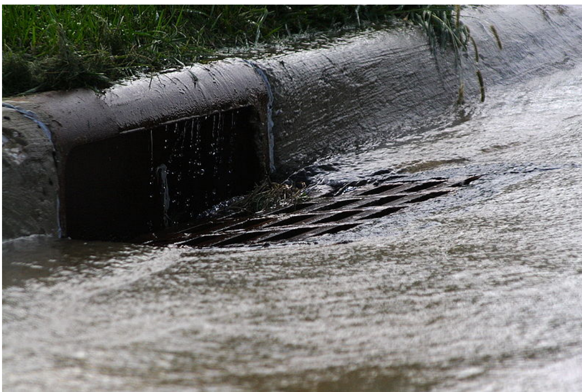
Figure 5.46: Storm Drain Curbside storm drain receiving urban runoff. Source: By Robert Lawton 53 via Wikimedia Commons
