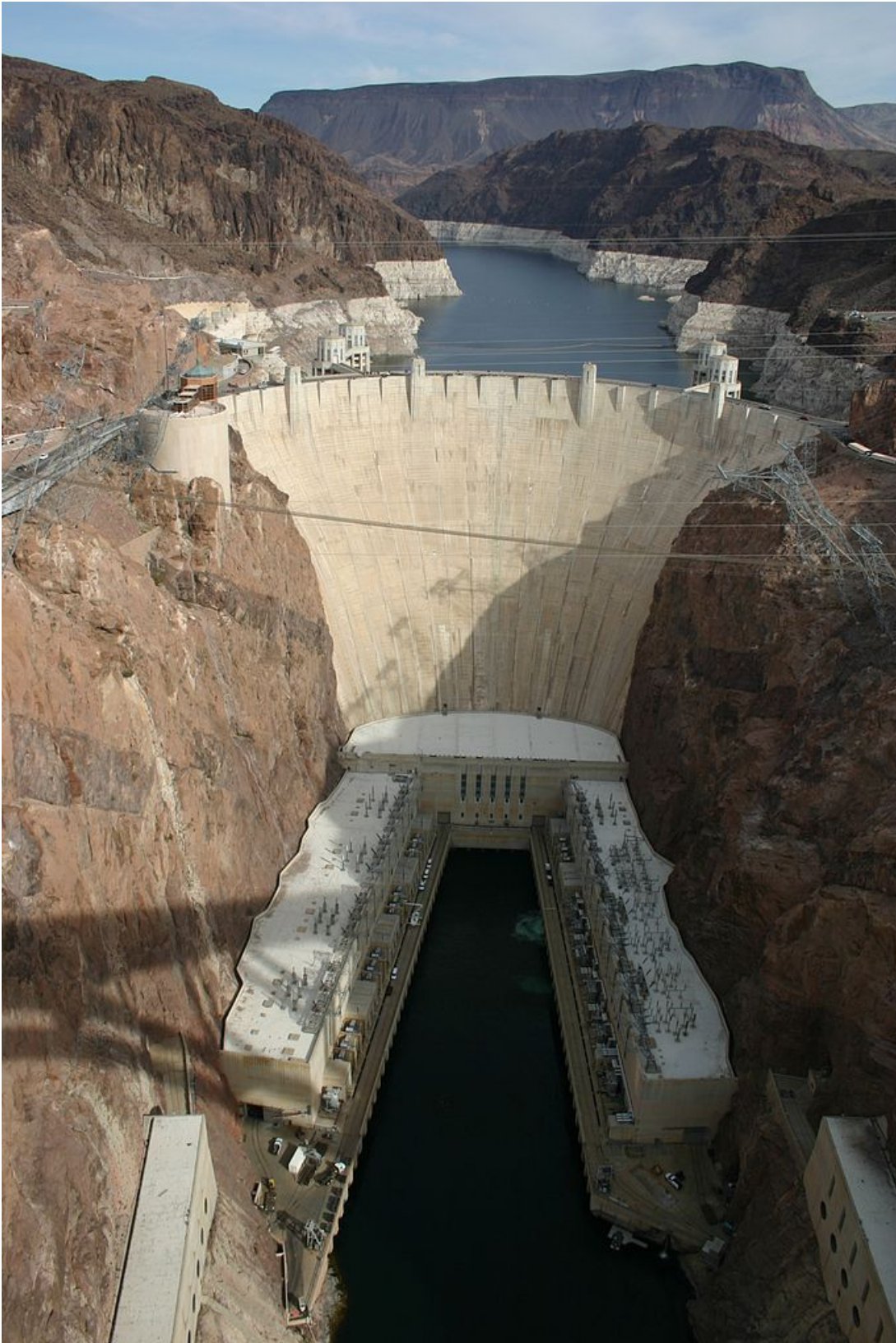
Figure 5.22: Hoover Dam, Nevada, U.S. Hoover Dam, Nevada, U.S.. Behind the dam is Lake Mead, the largest reservoir in U.S.. White band reflects the lowered water levels in the reservoir due to drought conditions from 2000 - 2010. Source: Cygnusloop99 26 at Wikimedia Commons
