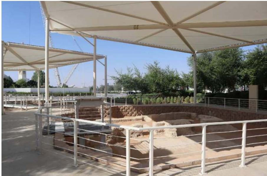
Figure 14: The shelters over the mosque and Falaj 1. (DCT Abu Dhabi, 2022)
