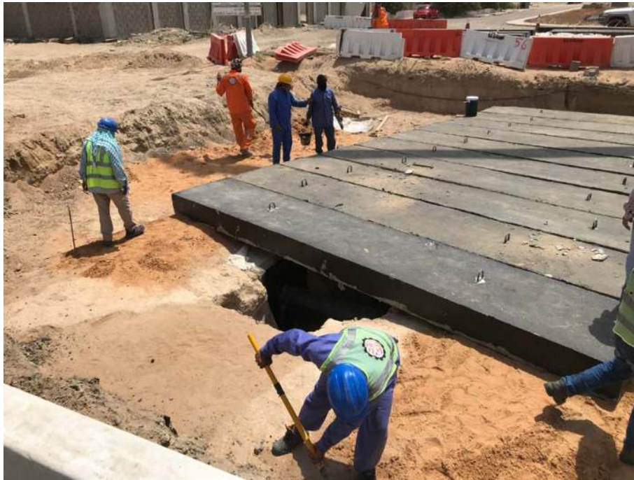
Figure 5: After documentation is complete, precast or cast in-situ slabs are used both to protect the aflaj and other significant archaeological features and to avoid future subsidence.
