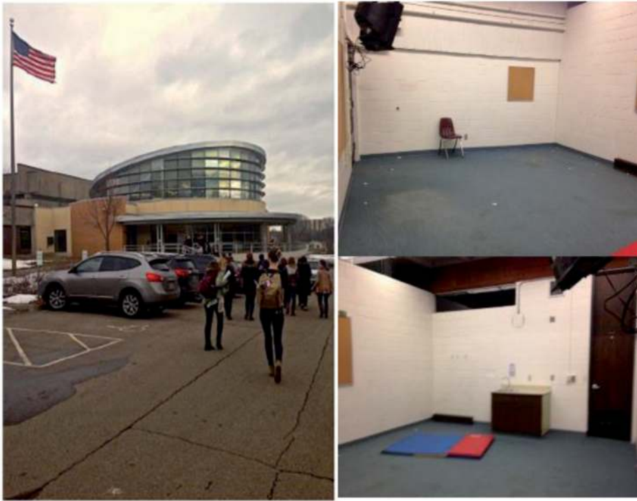
Figure 1. Bruce Vento School Exterior and former Calming Room Interior Condition (Source: Pictures by Author 1).
