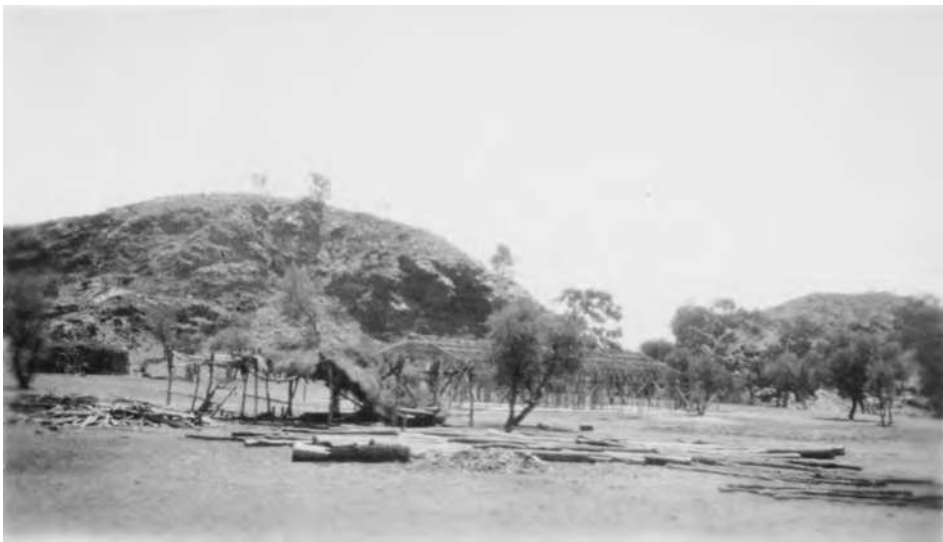
Figure 5: Building new dormitories at Iwaputarka (Jay Creek) 1929-32. See wiltja in foreground. NAA: 1928/59. Courtesy of National Archives of Australia.
