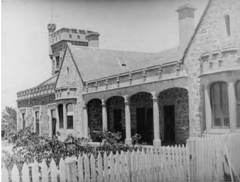
Figure 6: St Francis House on day of inspection for proposed purchase, 1947. NAA: A431/1. Courtesy of National Archives of Australia.
