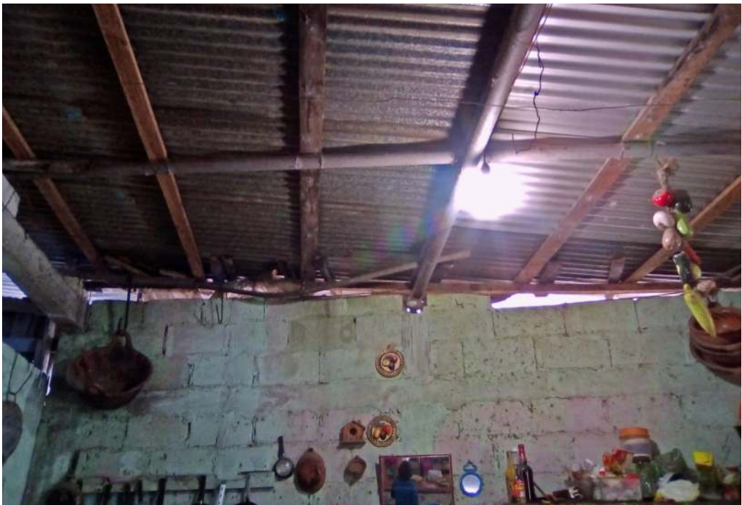
Figure 4.7. Decommissioned pipelines used as ceiling joists of a house in Emiliano Zapata, Papantla, Mexico, 2018 © Svenja Schöneich.
